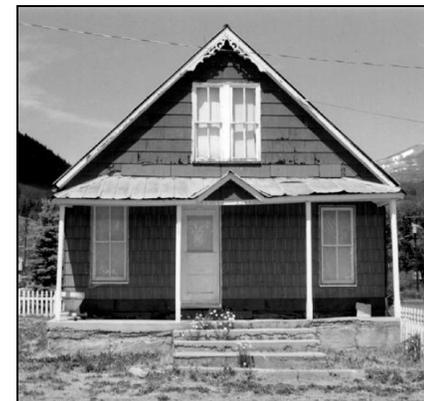
*Replacement materials should be similar in character to those used historically. This is an inappropriate use of materials. Coverings such as this obscure the original lap siding.*
