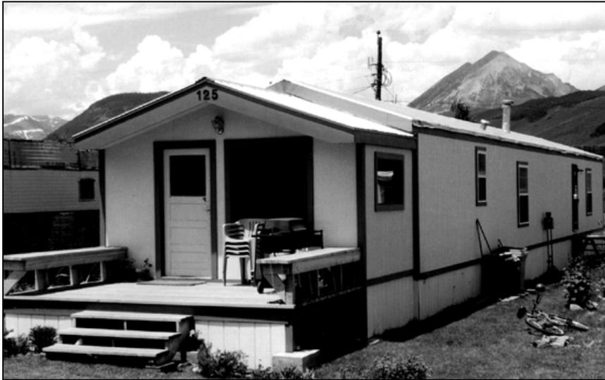
*Mobile homes should appear anchored to the ground. A skirt that screens the axle and tires and appears to be a foundation should be provided.*
