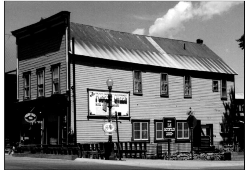
*The typical false front has a simple rectangular front façade, with a cornice at the top, used to conceal a sloped roof behind.*
