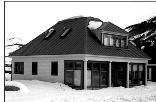
*The hipped roof house is characterized by the pyramidal shape of its roof.*
