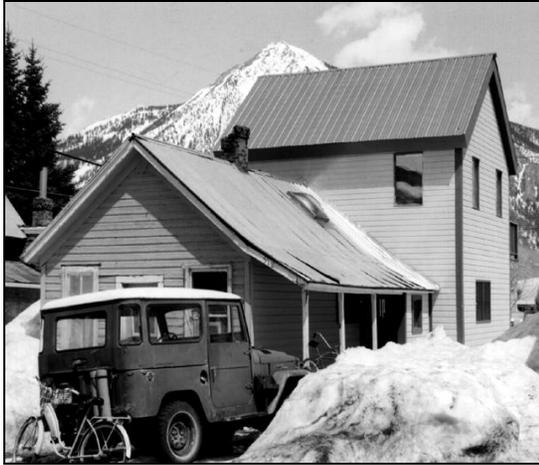
*New additions such as this create an appearance inconsistent with the historic character of the building, due to its height and change in roof peak orientation. This large addition should have been discouraged or separated from the original by a “connector” element.*
