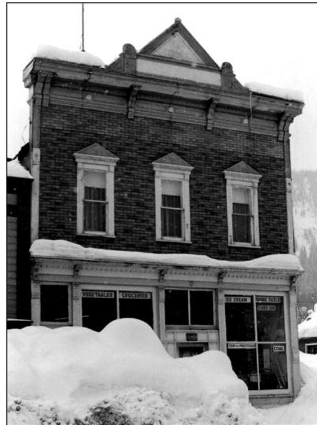
*Preserve original architectural detailing. Note that original metal siding is obscured by an imitation brick covering.*
